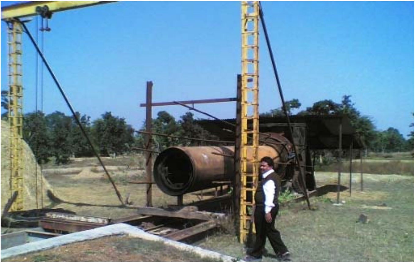
Water Proof Testing arrangement for Large Diameter Pipes
