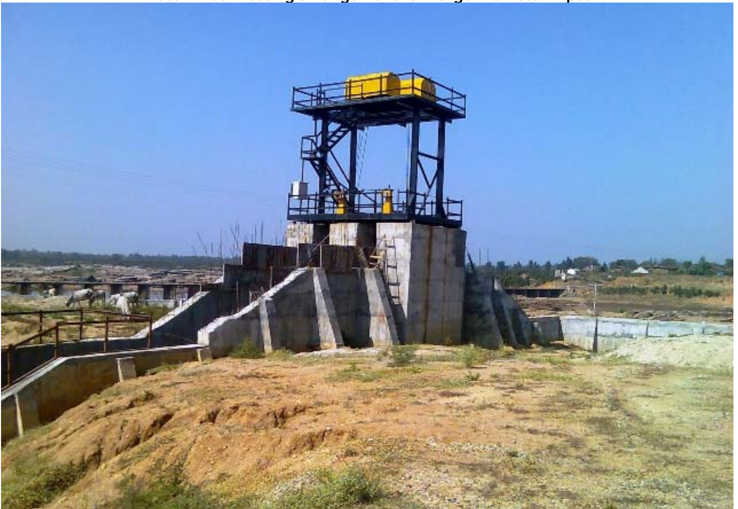
Head Work for Rajegaon Katee Lift Irrigation Scheme,
