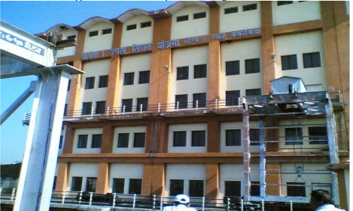
Pump house of Dhapewada Lift Irrigation Scheme.
