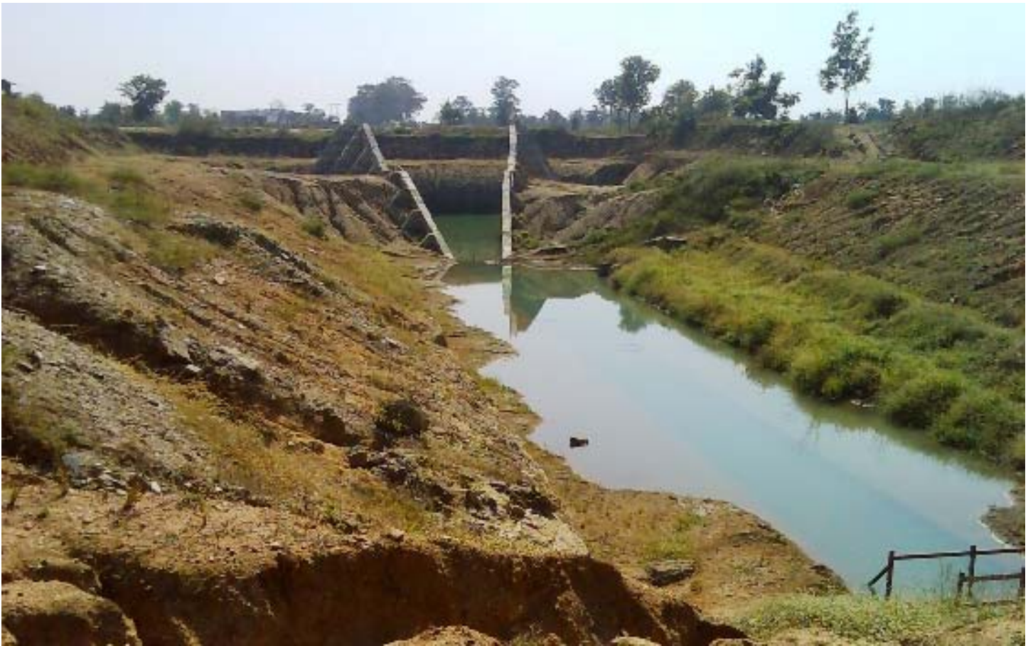
Approach channel to pump house for Rajegaon Katee Lift Irrigation Scheme,
