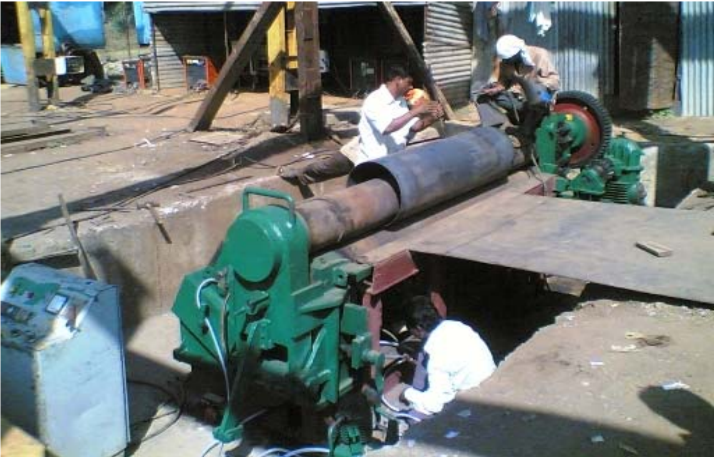
Bending of steel plates for fabrication of pipes
